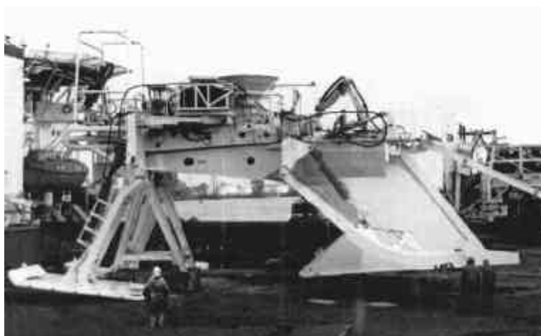
Figure 4 : ETPM's 4m Cable Plough
